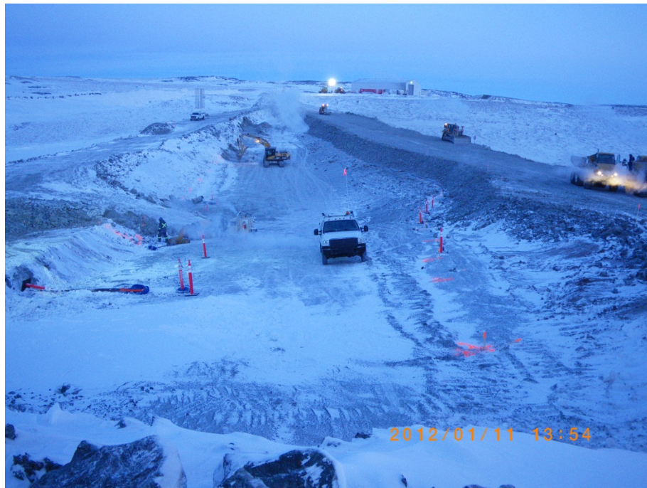
Photo 1: The 325 excavator is removing protective cover material along the downstream face of the key trench in the background. The temporary sump has been removed in the centre of the photo. The person standing next to ground temperature cables ND-HTS-060-28.8 and ND-VTS-060-KT. Ground temperature cables ND-VTS-040-KT and ND-HTS-040-31.5 have been cordoned off by traffic delineators in the foreground.
