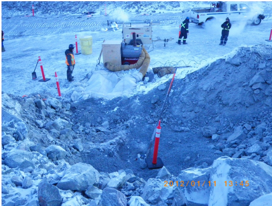
Photo 2: The traffic delineator, in the foreground, marks the location where ground temperature cable ND-VTS-060-KT comes out of the frozen fill. Ground temperature cable ND-HTS-060-28.8 has been severed, below the surface of the key trench. Hoarding is being applied to the frozen fill so enough cable can be exposed to allow for a splice to be made.
